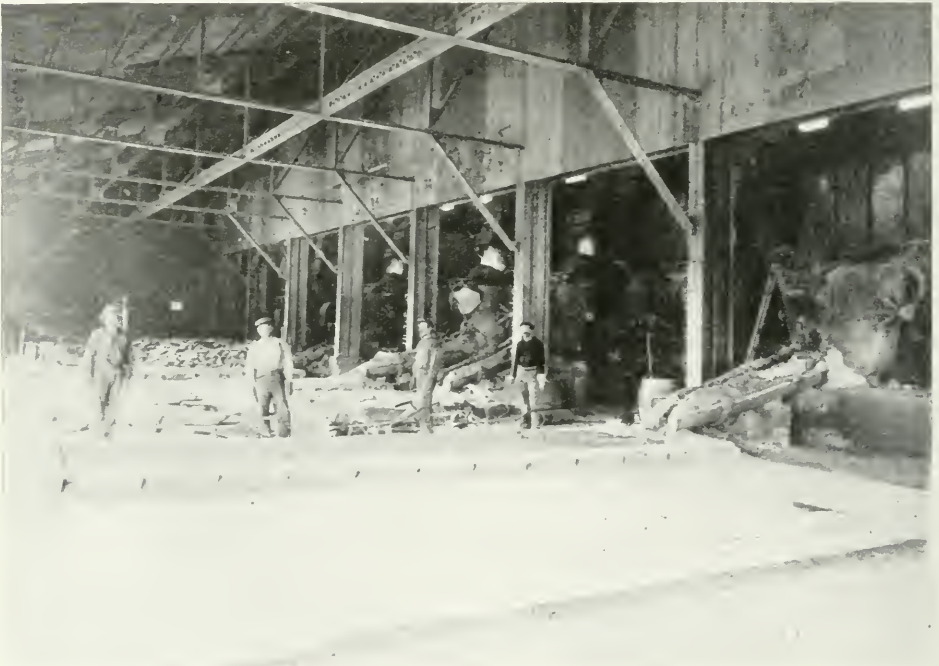
Fig. 75—Floor Moulds for Converter Matte, Canadian Copper Company, Copper Cliff.
